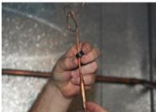
the SECOND piece to slide over the bulb is the PLATE
